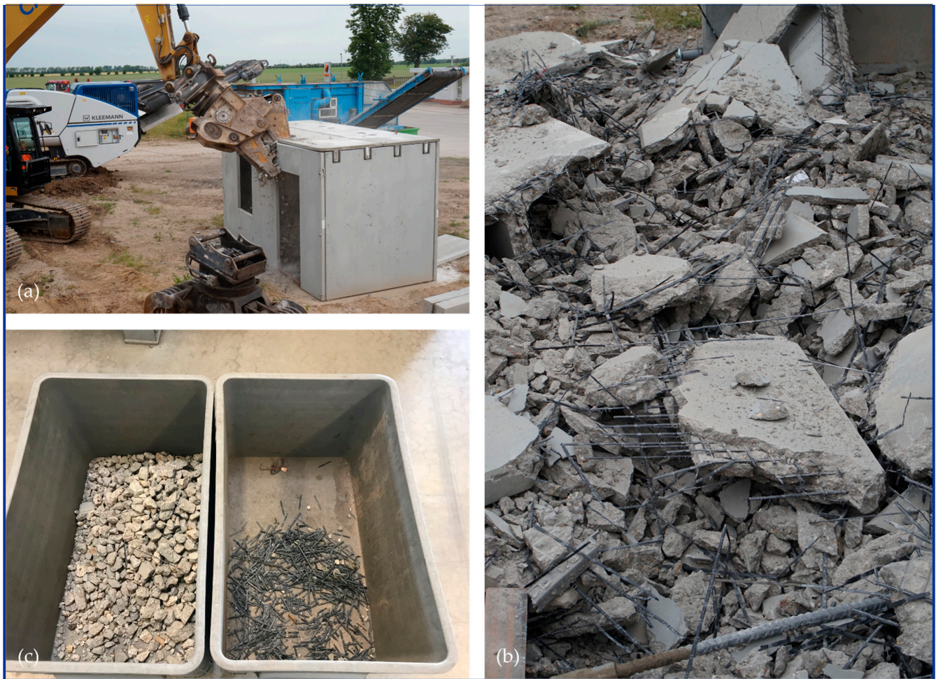
Figure 3. (a) Demolition with a concrete pulveriser, (b) pre-shredded demolition material made of carbon concrete, (c) result of camera-based sorting of carbon concrete containing demolition material, © Jan Kortmann.
