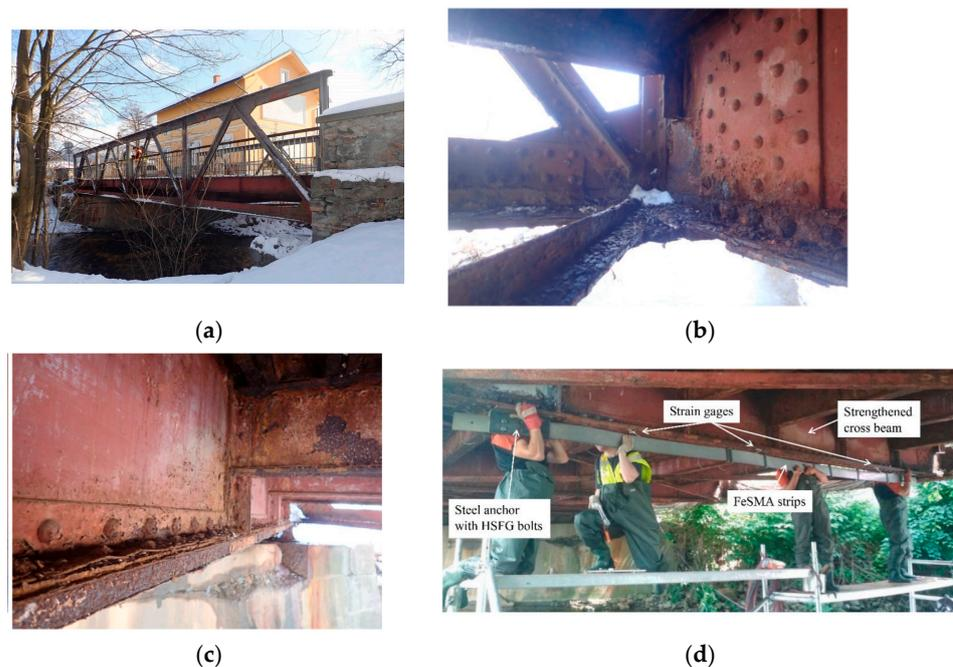
**Figure 20.** Historic steel road bridge: (a) 3D view; (b) damage point 1; (c) damage point 2; (d) installation of the Fe-SMA strips. Reproduced with permission from [112], Elsevier, 2021.
