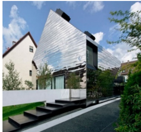
Figure 7. Textured stainless steel reflects a blurred picture of the surroundings that dynamically change according to position and time. House WZ/Bernd Zimmermann Architects, Germany, 2013. Source: Photography by Valentin Wormbs. https://www.archdaily.com/496803/house-wz-bernd-zimmermann-architekten/534ca246c07a80f3510001ab-house-wz-bernd-zimmermann-architekten-photo , accessed on 22 April 2023.
