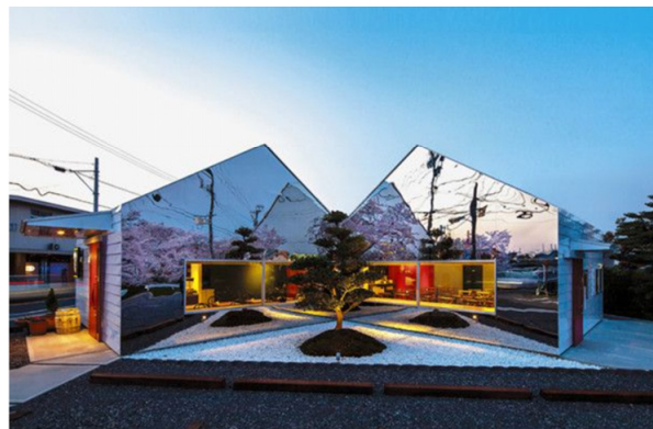
Figure 8. Polished stainless steel reflects the surroundings with glass windows showing the real exterior. Source: https://www.ribenbang.com/1038252/ , accessed on 22 April 2023.
