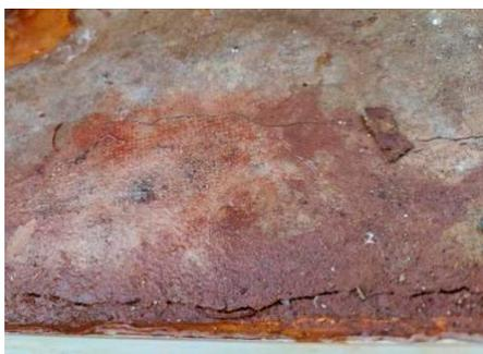
(a) Corrosion-induced cracks on the top plate
