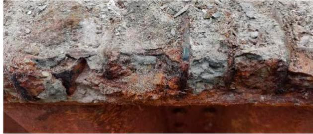
**Figure 9.** Corrosion of steel bars embedded in Beam A2.
