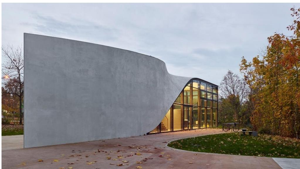
**Figure 1.** World’s first building constructed with carbon concrete (Photo: Stefan Mueller).
