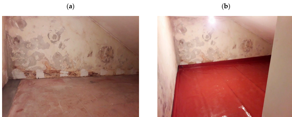
Figure 6. Placement of the Rn barrier membrane. (a) Floor before placing the barrier membrane; (b) Floor after placing the barrier membrane.
