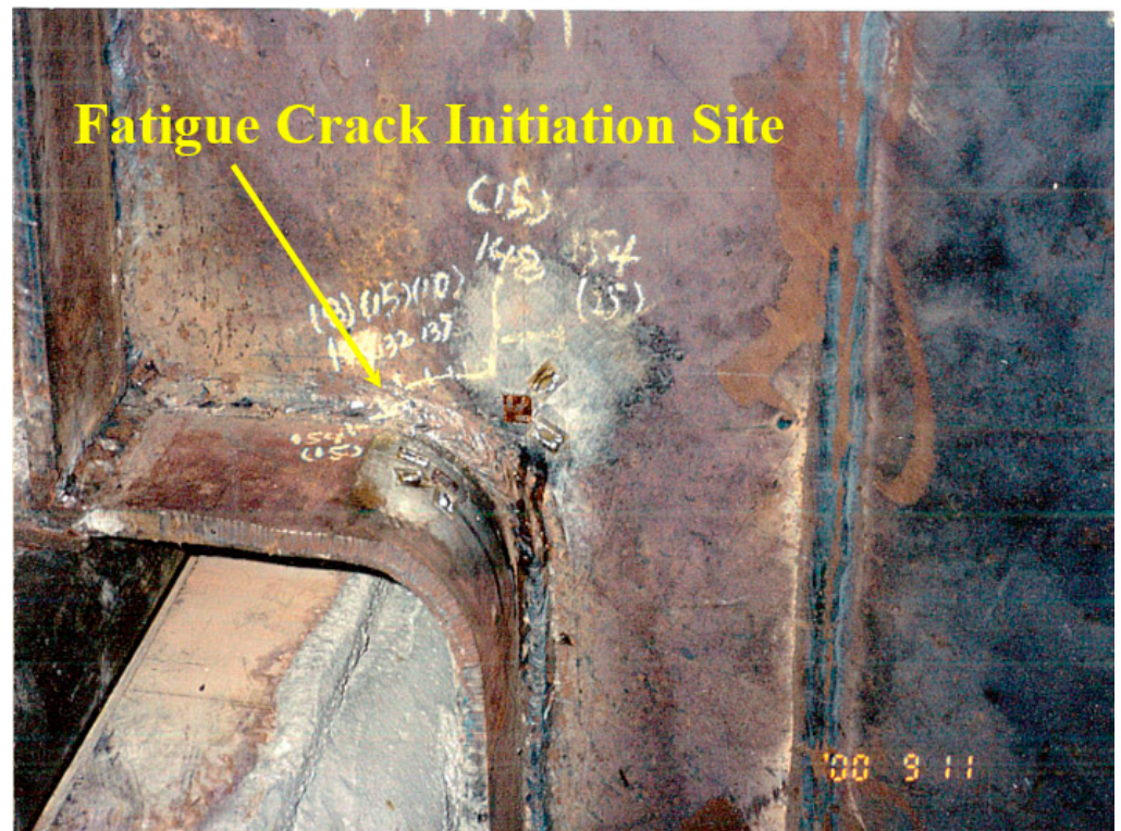
Figure 10. Cracks originated at the weld toe on the web.
