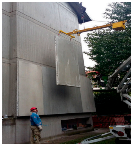
Figure 15. Installation of a prefabricated insulated element (i.e., EPS sandwiched between two layers of TRM) in a retrofit project in Italy (adopted from [43]).
