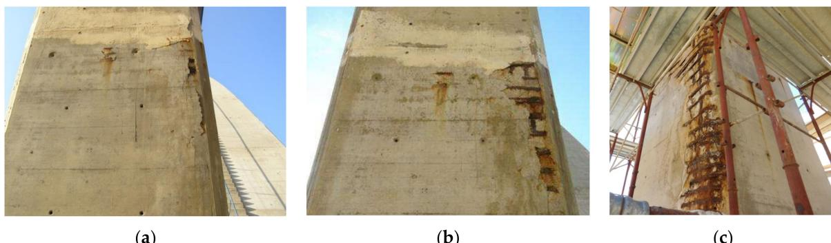
**Figure 4.** Propagation of corrosion of the reinforcement on the pier P3 in different periods: (a) 2006, (b) 2010; (c) 2017—shortly before repair.
