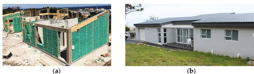
**Figure 1.** (a) SBT house under construction; (b) SBT house post-construction.
