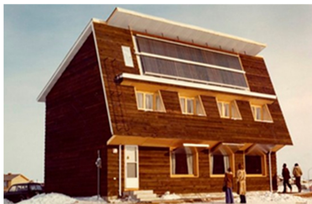
Figure 3. Saskatchewan Energy Conservation house designed by the Illinois U demonstrated passive technology in 1978 (Regina). Solar-exposed surfaces with large windows are inclined. Evacuated solar pipes are placed on the attic level. It was provided with an air-sourced heat pump and polyethylene-based heat recovery ventilator. Reprinted with the permission of Harold Orr.
