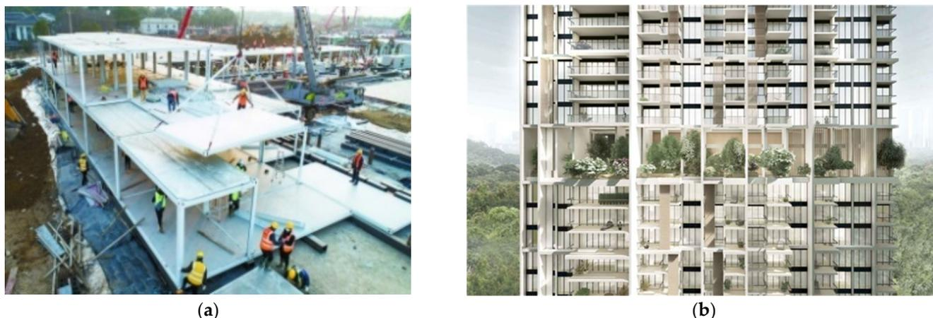
**Figure 1.** Mid-to-high modular construction: (a) Huoshenshan Hospital [7]; (b) 19 m tall towers [8].
