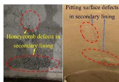
**Figure 3.** Tunnel second lining defect.
