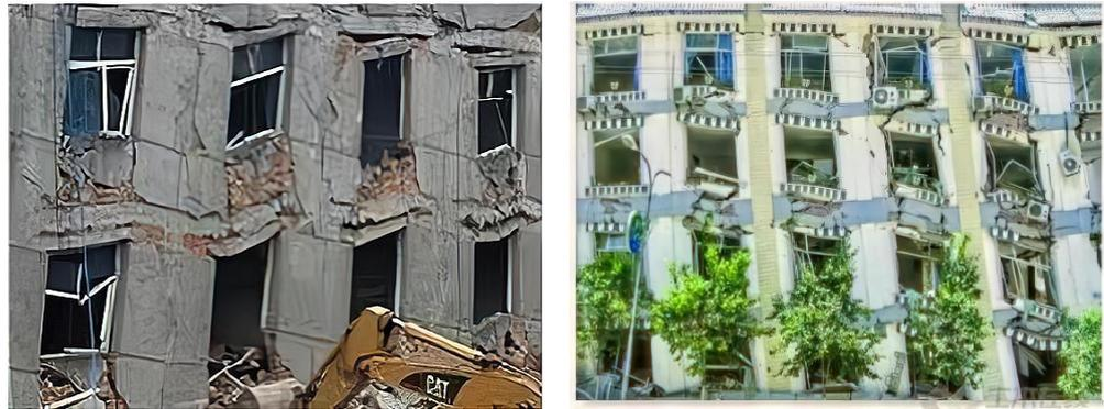
**Figure 3.** Damaged precast floor slab and spandrel in Ya'an, Sichuan, China.
