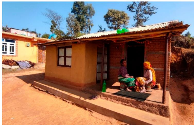
**Figure 4.** Houses built with Habitat for Humanity Nepal (HFHN) support allowed local designs with earthquake-resilient construction; note the horizontal ties in the walls (source: Sujit Maharjan, Habitat for Humanity, Nepal).
