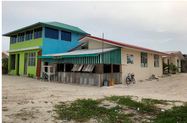
**Figure 1.** Houses in Dhuvaafaru with extensions and modifications; the house on the left was extended into a 2-storey structure (source: Iftekhar Ahmed, University of Newcastle, Australia).
