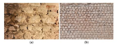
Figure 8. Texture of the masonry, after the restoration of the belfry (a) and of the nave wall (b).
