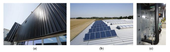
**Figure 10.** Solar wall that heats the assembly plant (**a**), a system of solar and photovoltaic panels on the roof (**b**) of building B-02, Smart Building Center–W.P.I.P. reprinted with permission from ref. [72] and the ventilation room (**c**) of building B-05 Nowy Targ [photographs taken by Kirschke, P.].
