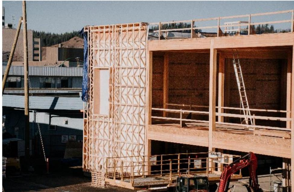
**Figure 1.** Wood Innovation Research Lab glulam post and beam structural system with vertical truss wall panel to be insulated on site.
