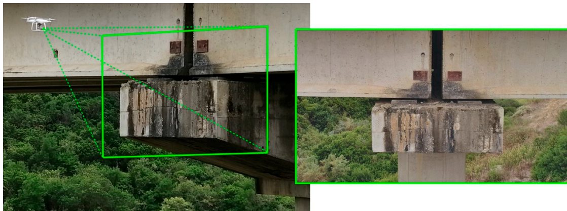
Figure 6. Visual inspection of the side of the structure by RPAS in manual mode.
