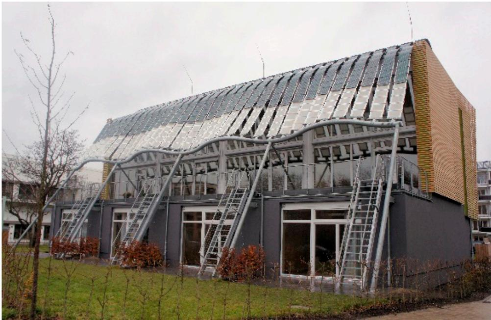
**Figure 11.** Solar electricity generating thin-film system independent of the building (photo by W. Celadyn).
