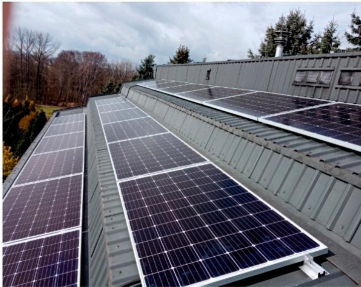
**Figure 8.** Stepped roof with PV monocrystalline photovoltaic panels installed at the recommended angle of  $15^\circ$ . Location:  $49^\circ 57'$  N,  $19^\circ 55'$  E (photo by W. Celadyn).
