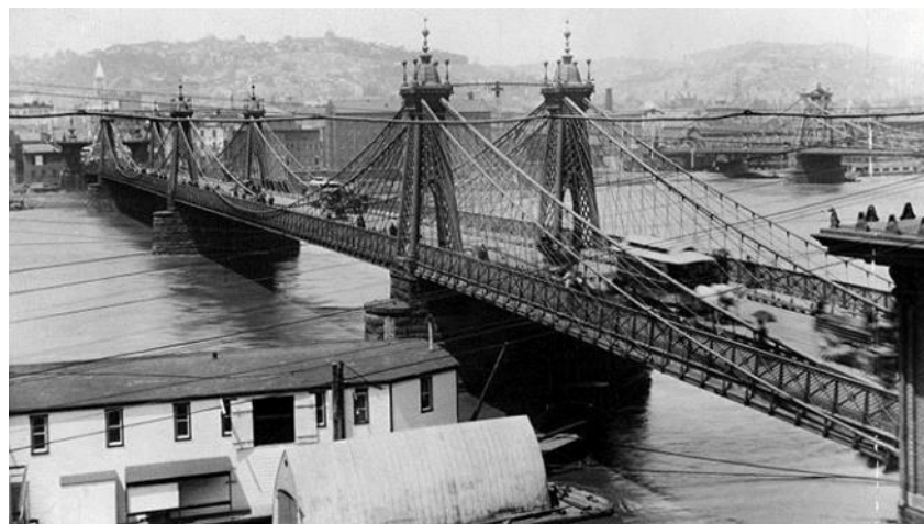
Figure 16. Monongahela Bridge, Continuous Span Compensation Suspension Structure. Designed by Roebling. Pittsburgh. 1846. Source: The Carnegie Library of Pittsburgh.
