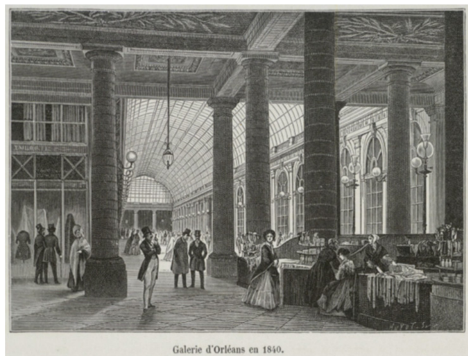
Figure 3. Galerie D'Orléans. Iron and glass architecture system for vaulted structures. Fontaine and Rohault, Orléans, France in 1840. Source: Brown University Center for Digital Scholarship engraving of the collection "Paris, capital of the s. XIX".
