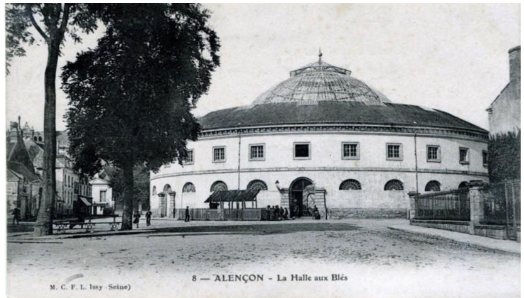
Figure 8. La Halle aux Blés. Photograph showing the replacement of the old wooden structure of the dome with iron and copper ribs according to the design of Bellangé and Brunet in Paris 1811–1820 by Bellangé. Source: Extract from Dictionnaire des rues et monuments d’Alençon (Alain Champion, Éditions Cénomane, 2003).
