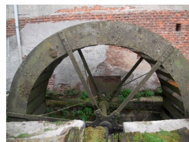
Figure 5. The overshot water wheels of the Riviera mill: (a) Before the renovation (Courtesy of Arch. Roberto Olivero, 2004); (b) after the renovation.
