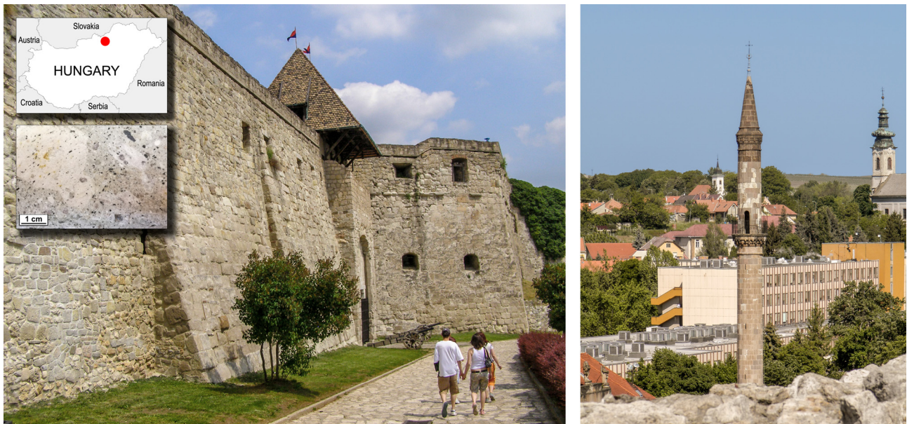
Figure 1. Examples of the historical usage of tuffs in the town of Eger: the Medieval castle and the Ottoman minaret. The insets show the location of the study quarry sites (a few kilometers apart) and the macroscopic appearance of Demjén tuff used in the monuments.
