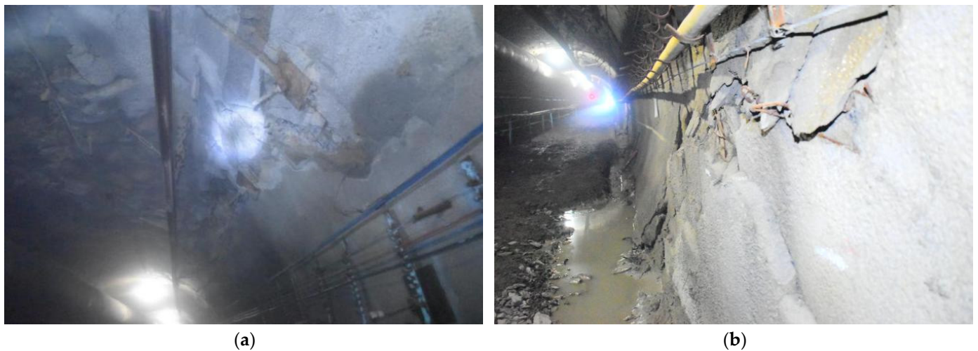
Figure 4. Damage characteristics of west wing transportation roadway. (a) Roof fracture. (b) Cracking on side of roadway.
