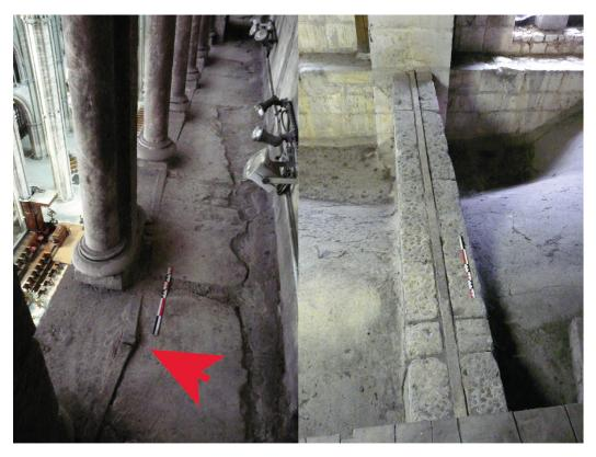
**Figure 2.** (left) Triforium chain (red arrow). View of the north side in the 2nd bay, (right) Attic tie rod TN4.
