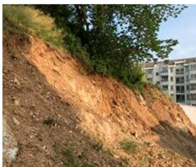
**Figure 4.** Failure scene of a soil–rock slope in Zhenjiang.
