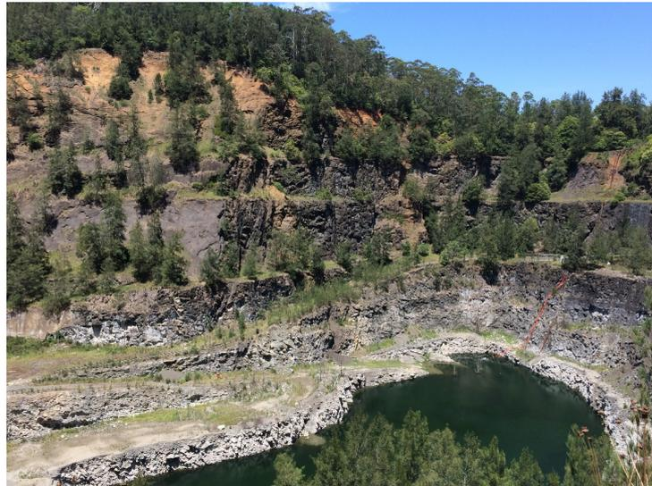
**Figure 3.** High-angle surge layers in the southern face of Hornsby Quarry: an important feature of diatremes at the macro- to mesoscale. Benches are up to 30 m in height.
