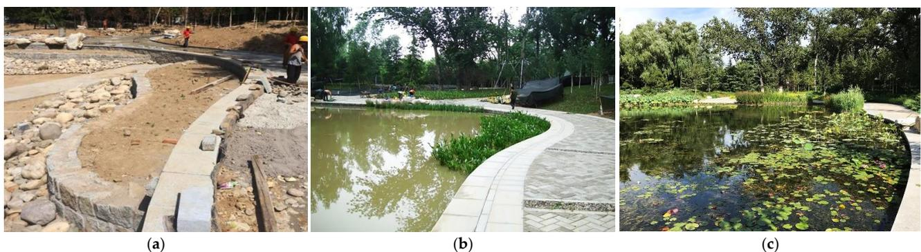
**Figure A2.** (a) Construction of “multilevel” revetments and lakebeds at pond 4; (b) aquatic macrophytes were planted in the “multilevel” pond revetments and lakebeds of pond 4, forming a “multilayer” plant configuration in the second experimental year, and the water quality was relatively poor in the initial stage of remediation; (c) aquatic macrophytes grew well, and the water quality was greatly improved in the third experimental year.
