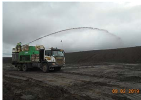
Figure 6. Hydroseeding application on post-coal-mining landscapes.
