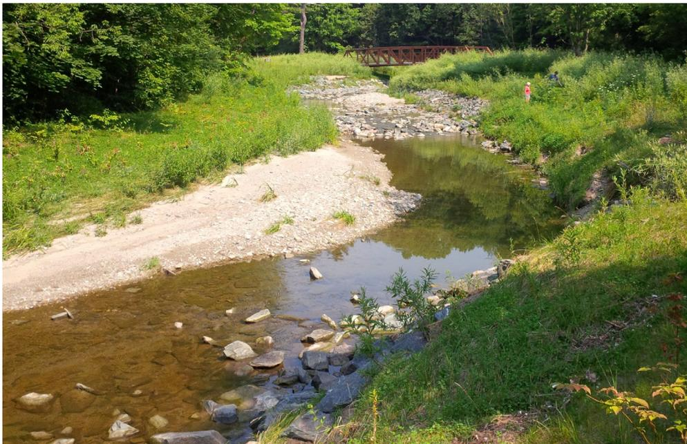
**Figure 3.** Photograph of restoration site July 2013, approximately 18 months after construction. Note the rocky riffle upstream of the pool in the middle of the frame and the point bar largely formed from deposited sand and gravel. Flow is from top to bottom.
