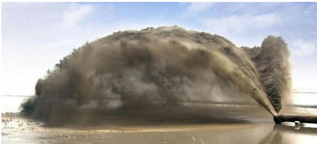
**Figure 1.** A photo showing the filling process of dredged soil during a land reclamation project.
