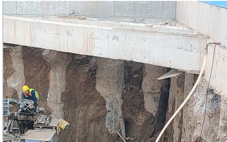
Figure 4. On-site construction of corner braces.
