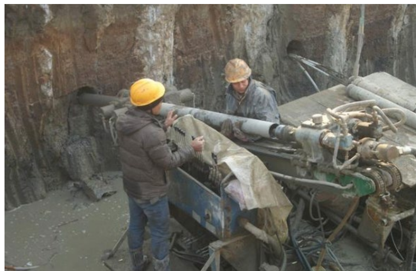
Figure 3. Drilling construction of anchor cable.
