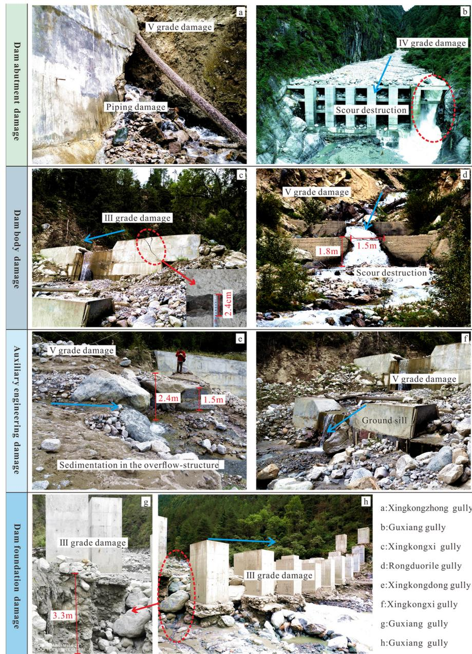
Figure 4. Damage types for check dams subject to glacial debris flow.
