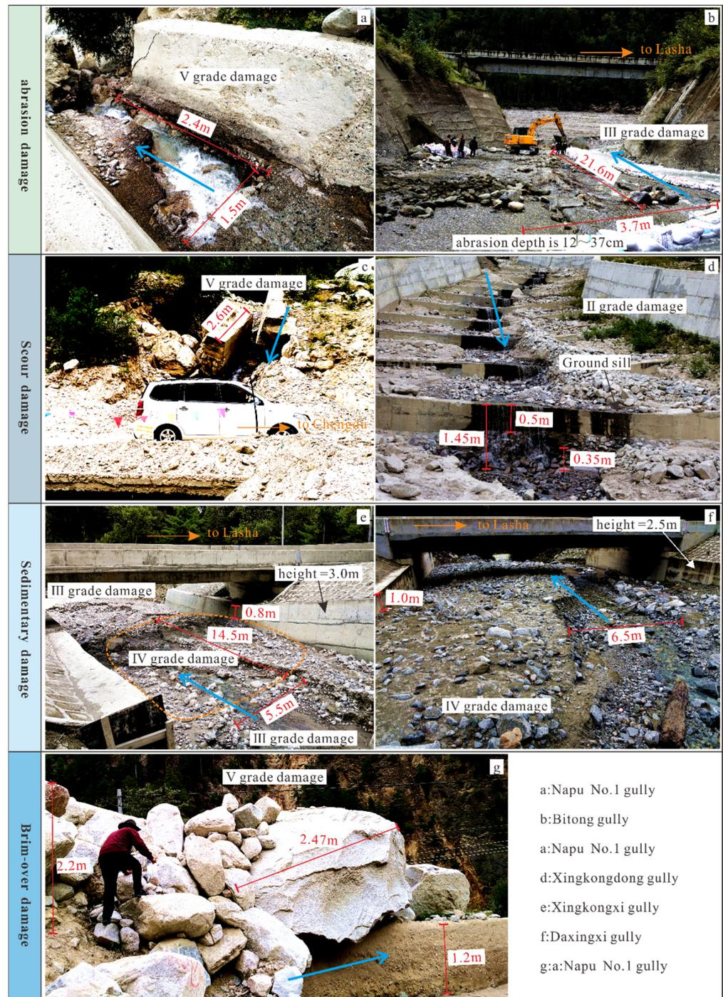
Figure 3. Damage types for drainage channels subject to glacial debris flow.
