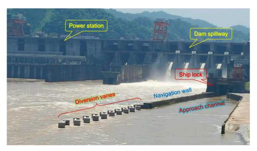
Figure 14. Actual layout of diversion vanes in the Wuqiangxi hydro-junction.
