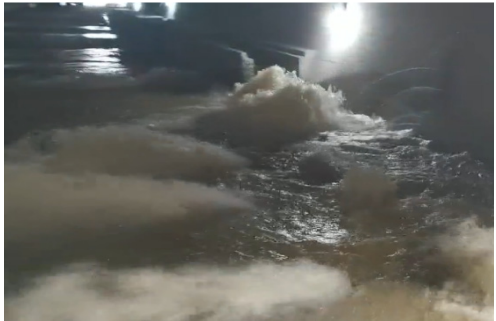
Figure 7. Water inrush in the tunnel after initial treatment.
