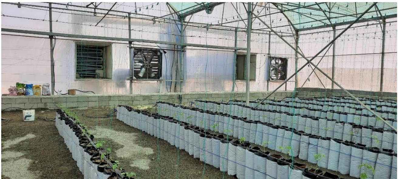
Figure 6. The position of ventilation fans installed in the seawater greenhouse.
