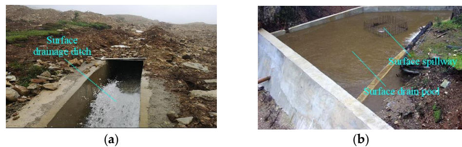
Figure 10. Surface flood control and drainage systems within the Plan mine sinkhole. (a) Surface flood control by intercepting ditch; (b) surface spillway.
