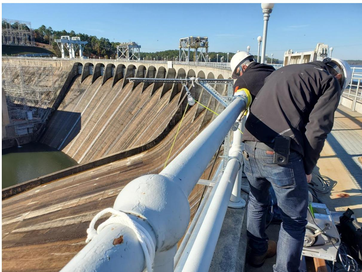
**Figure 5.** Photographs show crawler with GPR being lowered onto spillway after implementation of 1 m boom.
