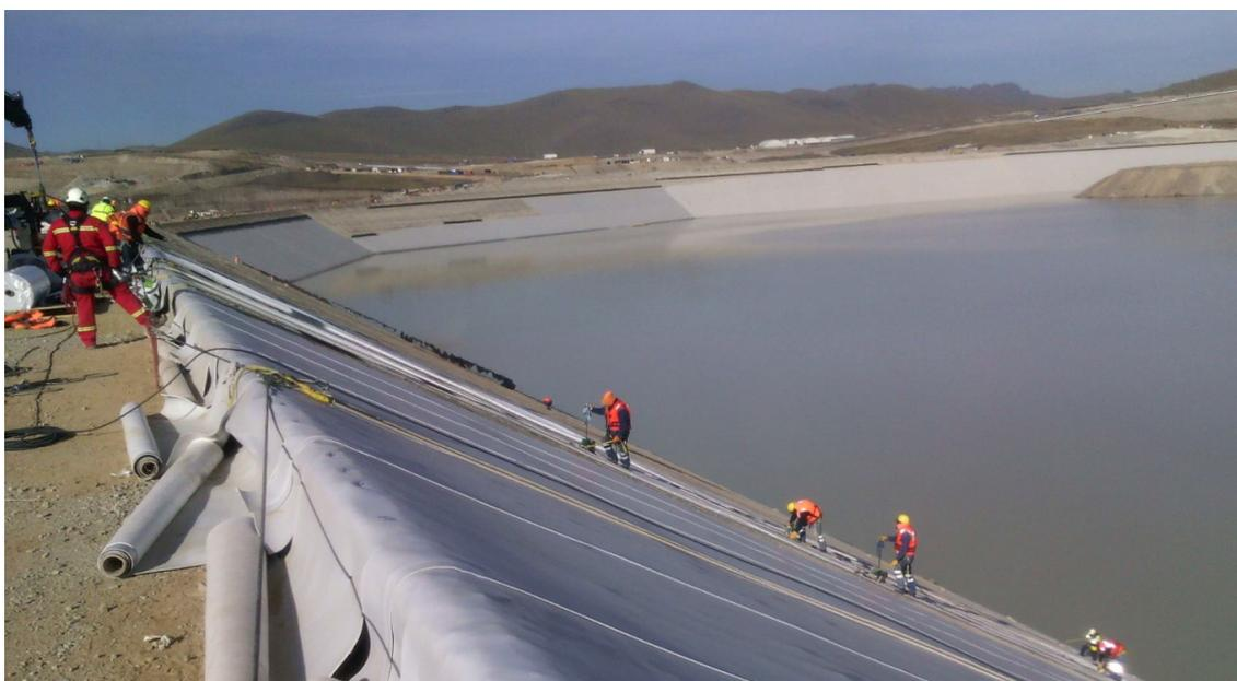
**Figure 13.** Geomembrane installation—typical construction activities, 2H:1V dam slope—Peru.
