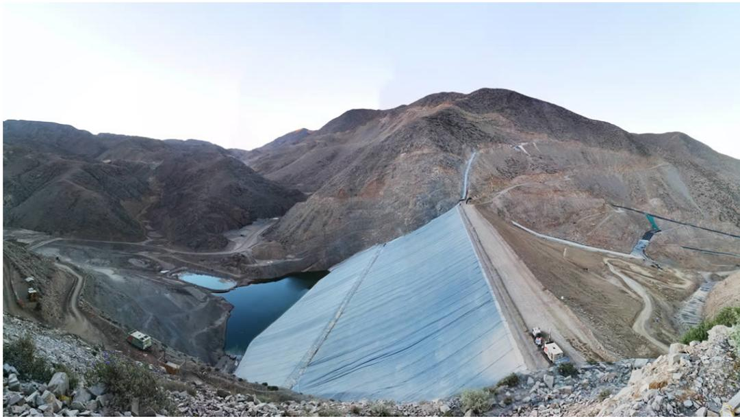
**Figure 23.** Panoramic view—mine waste rock dam upstream face waterproofing construction detail—TSE, Peru.
