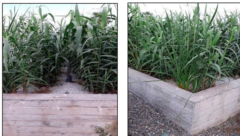
Figure 1. An overview of the vertical subsurface flow system (VSSFs) constructed wetland (CW) at ExpA_1.
