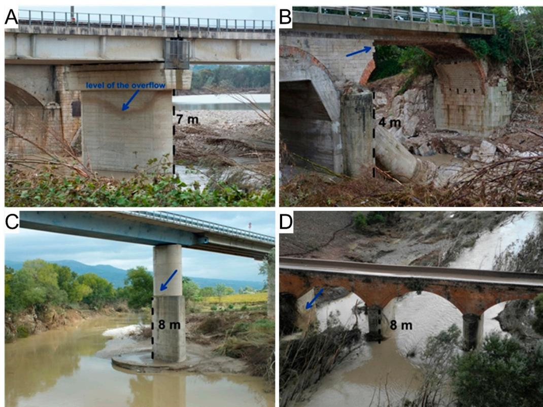
**Figure 10.** River stage during the overflow of the Tammaro and Calore rivers and Tammarecchia torrent, evidenced by flood marks on bridges, in different places across the Benevento province: (A) The Tammaro river in the industrial area (ASI) of Benevento; (B) the Tammarecchia torrent in Circello; (C) the Calore river in Paupisi; (D) the Tammaro river southwest of Circello.
