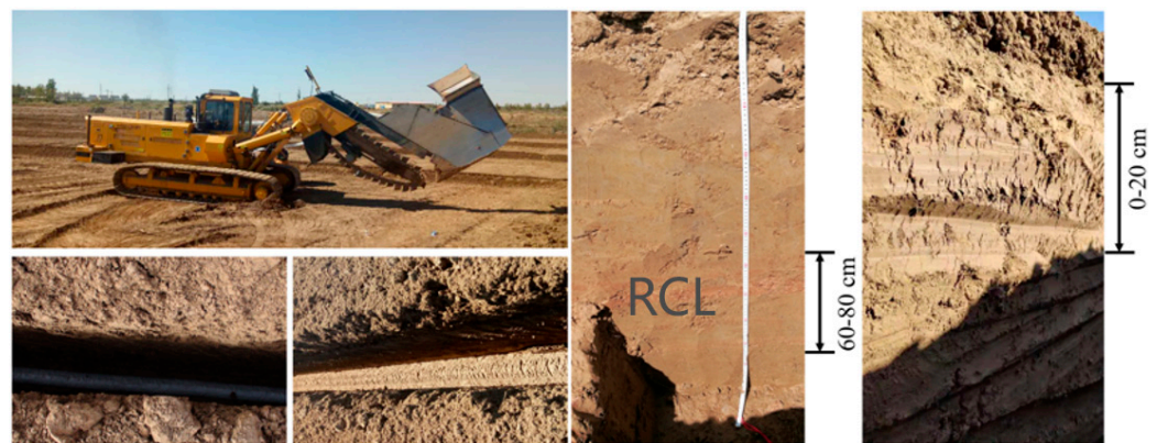
Figure 1. Buffer lines of pipeline laying and distribution of the red clay layer (RCL).
