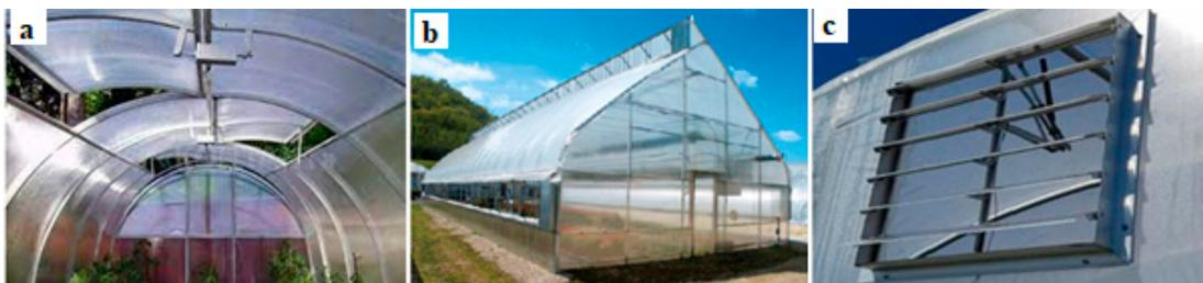
**Figure 2.** Different types of greenhouse openings: (a) roof vents; (b) ridge vents; (c) side vents.
