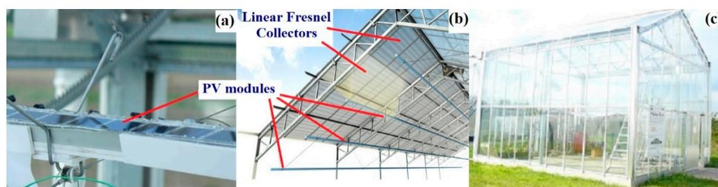
**Figure 10.** (a) The PV modules of the system; (b) the linear Fresnel collectors of the system; (c) the Fresnel greenhouse (The Netherlands). Reprinted with permission from Ref. [103]. Copyright 2011 Elsevier.
