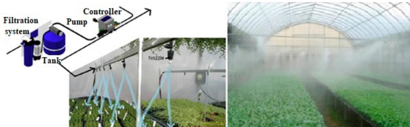
**Figure 7.** Schematic of cooling by a fogging system. Reprinted with permission from Ref. [97]. Copyright 2019 Elsevier.
