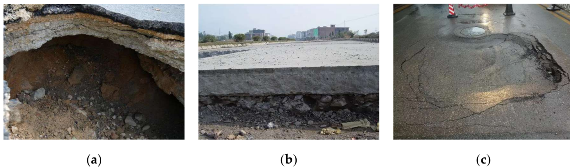
Figure 1. Common road diseases. (a) Subgrade debonding; (b) Subgrade weakness; (c) Road subsidence.
