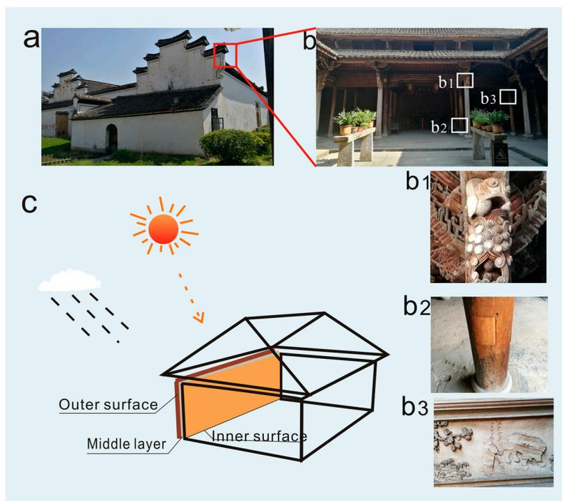
**Figure 1.** Damage and repair of typical ancient wood buildings (a: ancient wooden building exterior view; b: ancient wooden building interior view; b1&b2: damaged wood carving; and b3: repaired with fresh wood; c: The specific positions for taking samples).
