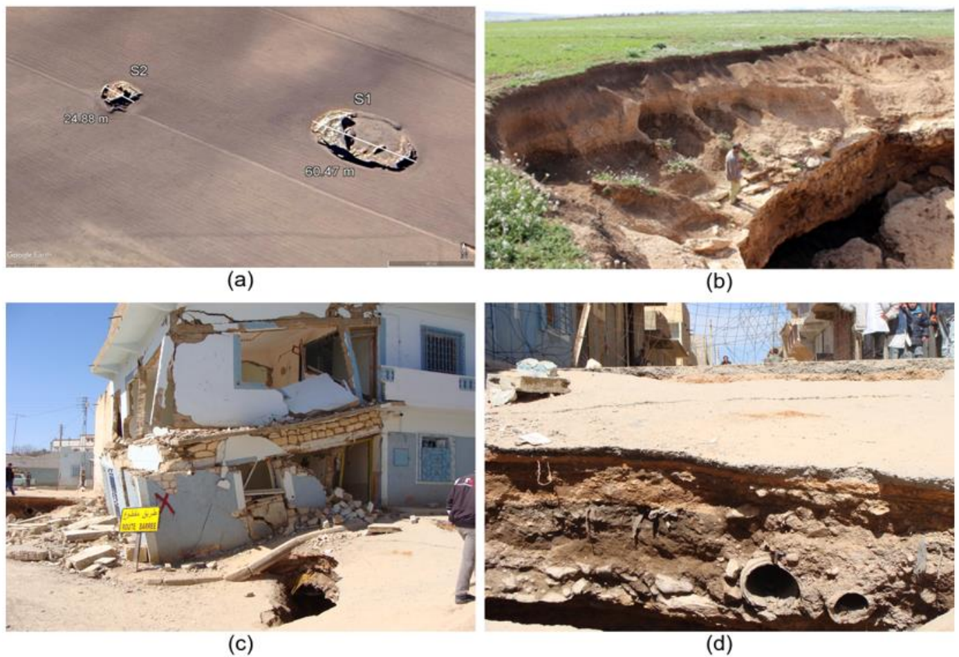
Figure 3. Sinkhole example images: (a) Draa-Douamis sinkholes 1 and 2 collapsed with a diameter of 66.47 and 24.88 m, respectively (location: see Figure 1—sinkhole sites; date: during 2004); (b) example of sinkhole diameter enlargement in surface; (c) Harkat Bouziane sinkhole collapsed in the city with a diameter of ~50 m and height of 2 m (location: see Figure 1—sinkhole sites; date: February 2009), destroying infrastructure; and (d) damage created by a sinkhole event (i.e., sewer network and roads broken).
