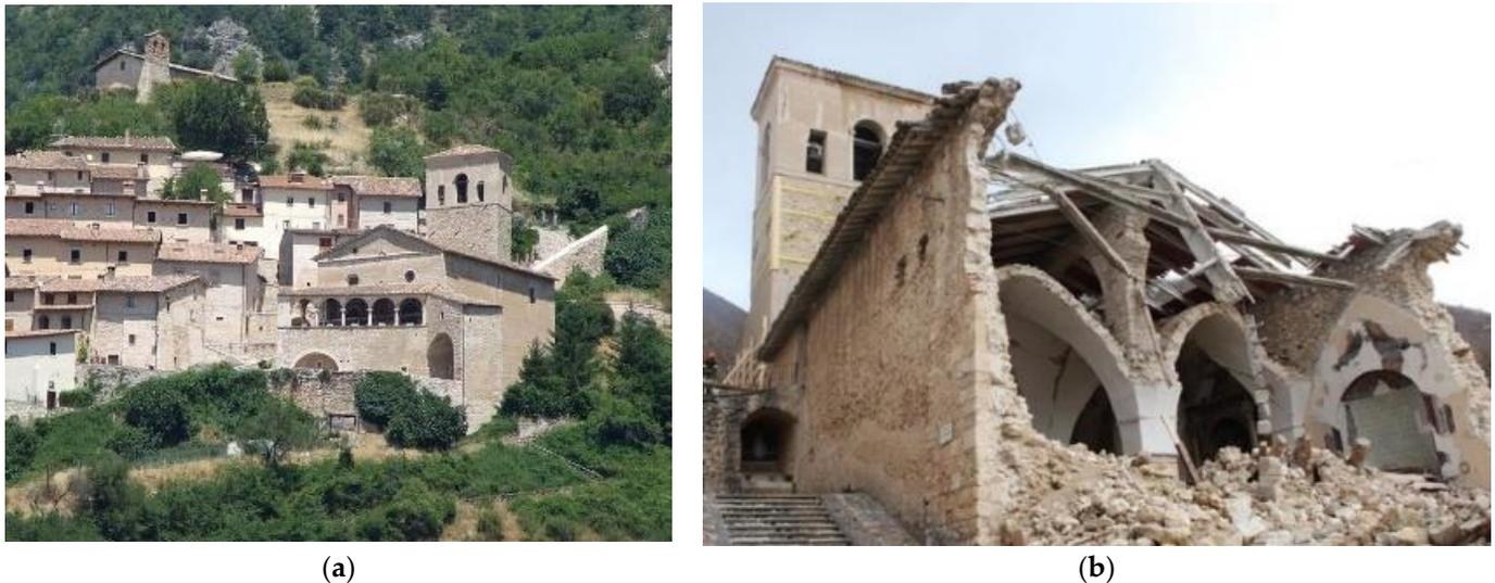
**Figure 3.** (a) The church of Sant'Andrea, with its bell tower and portico, prior to the 2016 earthquake. (b) The church following the collapses related to the 2016 earthquake.
