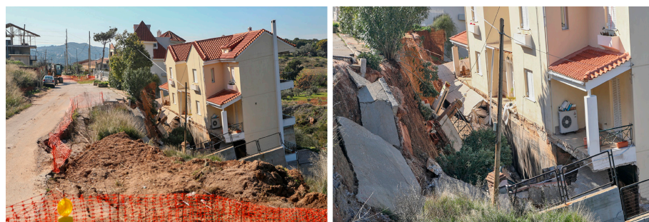
Figure 2. Residential building subsidence occurred at the beginning of September 2022 in Neos Voutzas following an intense rainstorm. The images are sourced from the archive of the Hellenic state television ( https://www.ertnews.gr/tag/neos-voutzas/ , accessed on 3 August 2023).
