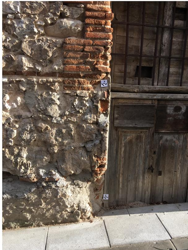
**Figure 11.** Example of the precision marks used.
