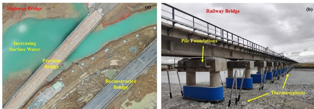
Figure 14. Countermeasures used by the (a) highway and (b) railway downstream to cope with flowing water drained from Salt Lake.
